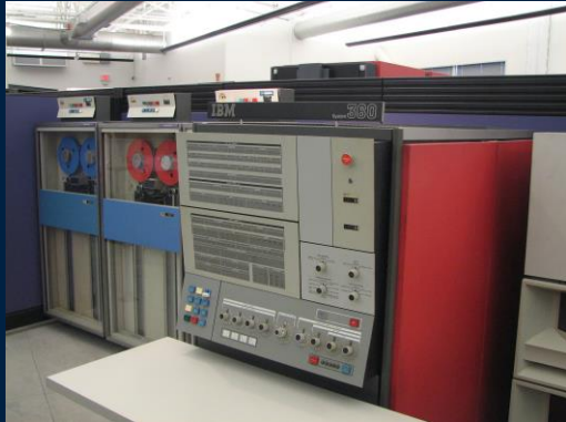
Erik Pitti - Flickr: IBM System/360 Mainframe CC BY 2.0
