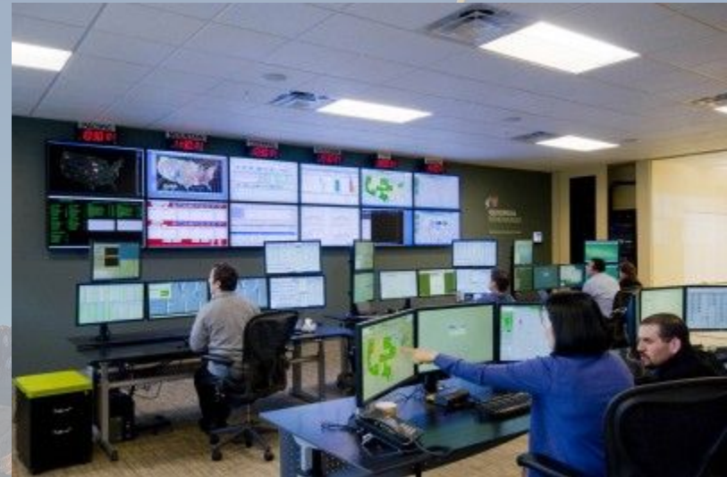
Iberdrola Renewables Control Room
